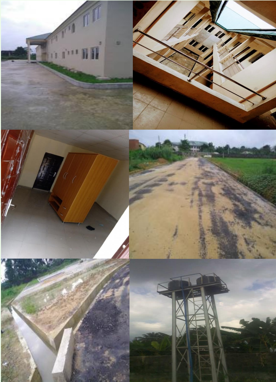
Figures 13 (e): Completion of construction, furnishing, landscaping and provision of water reservoir, RHCC, CNES & Construction of road and drainage network, 2019.
